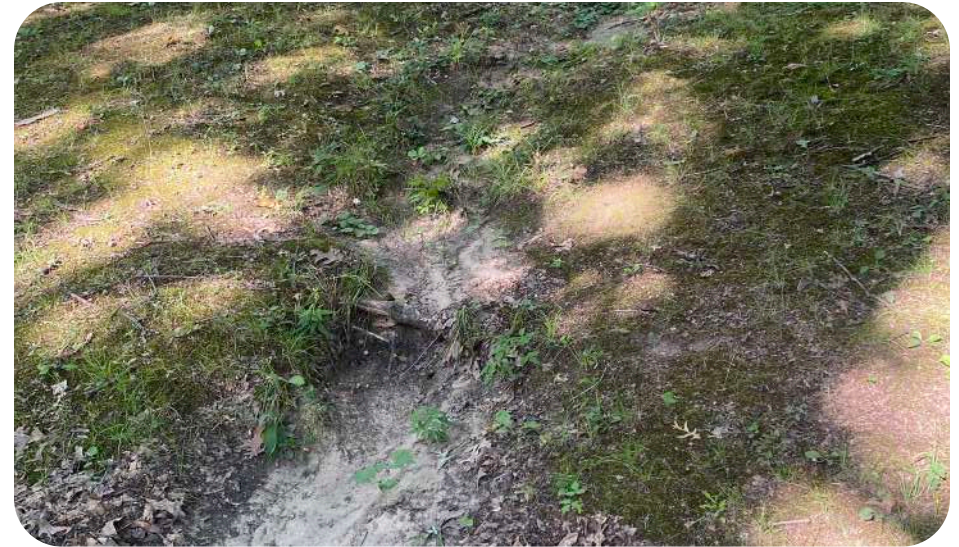
Figure 101. Existing soil erosion
