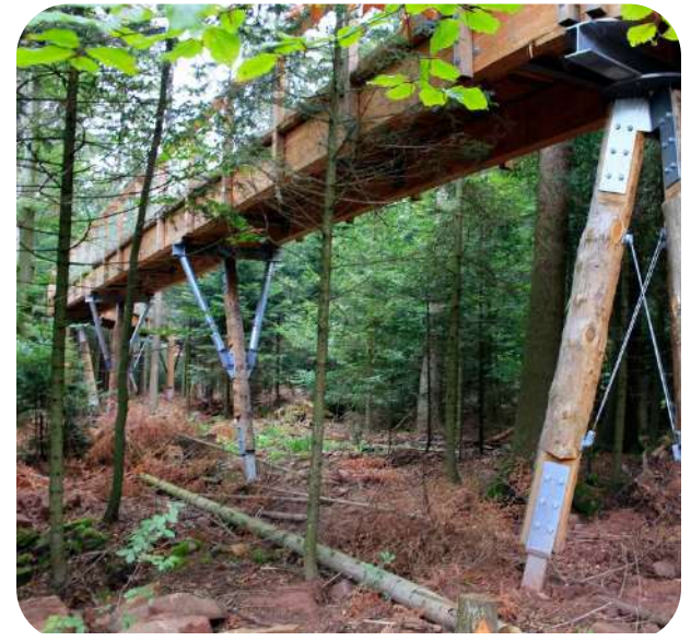
Figure 56. Low impact foundation structure
