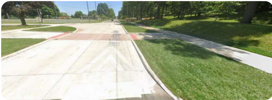
Figure 12. View looking east on W. Ewing Avenue
