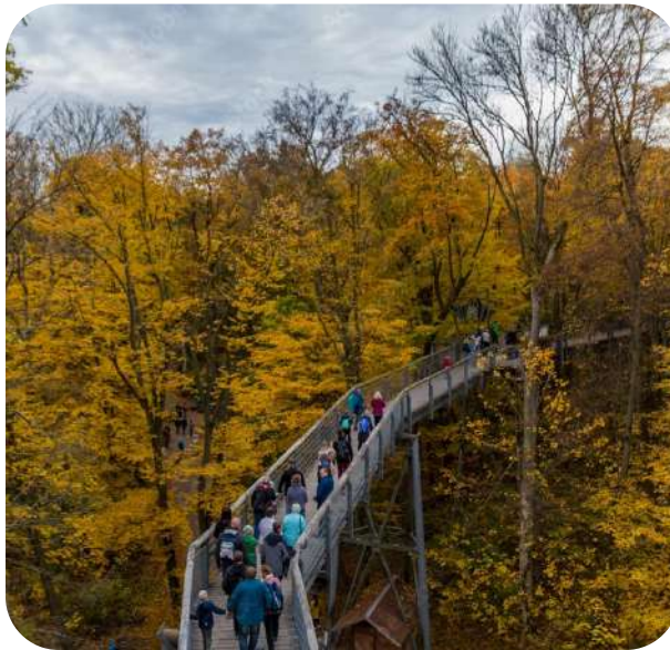
Figure 55. Lightweight steel structure
