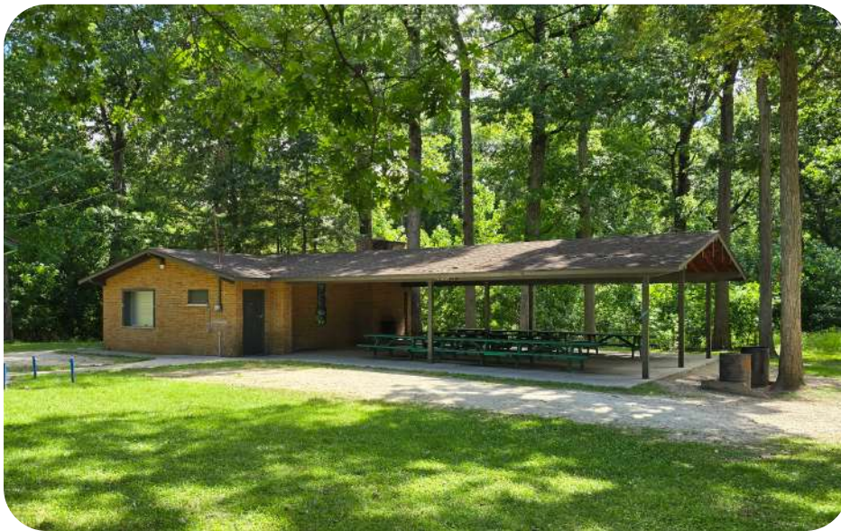
Figure 92. View of existing Pavilion 1
