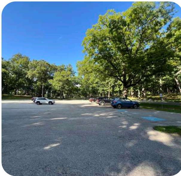
Figure 22. Very gentle slopes at parking lot area
