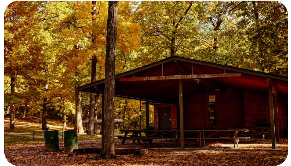
Figure 93. View of existing Pavilion 1
