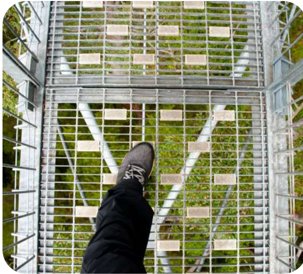
Figure 53. Metal structure and grate
