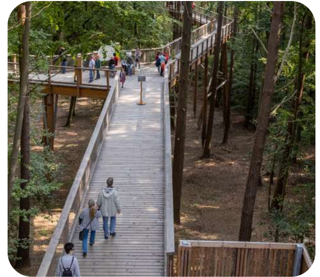
Figure 54. Timber decking and guardrails
